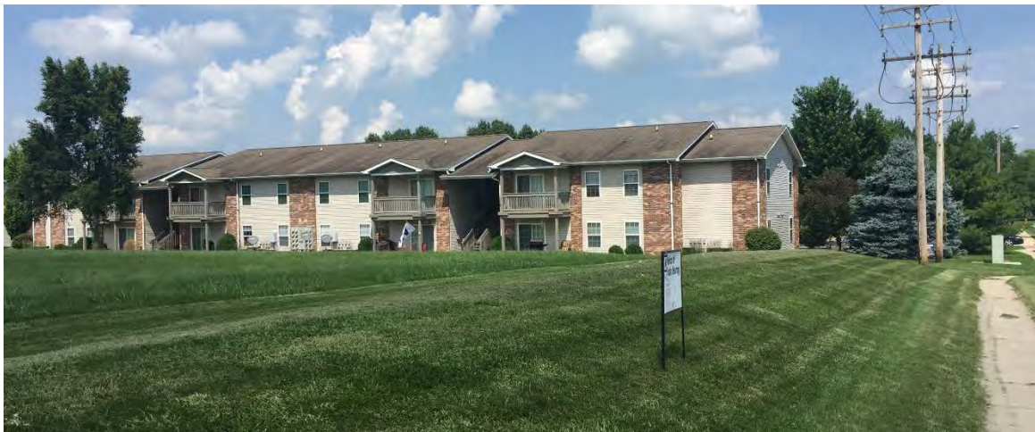
East property line: Stone Ridge Square Apartments
