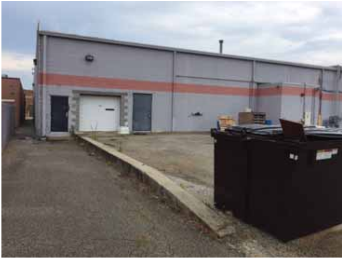
Figure 4. Rear of storefront.
