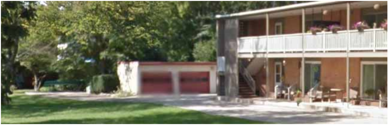
Figure 1. Dwelling and garage at 717 S. Broadway Ave.
