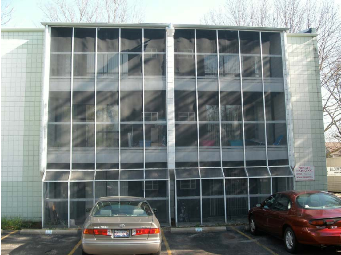
BUSEY COURT APARTMENTS – TYPICAL EXISTING BALCONIES
