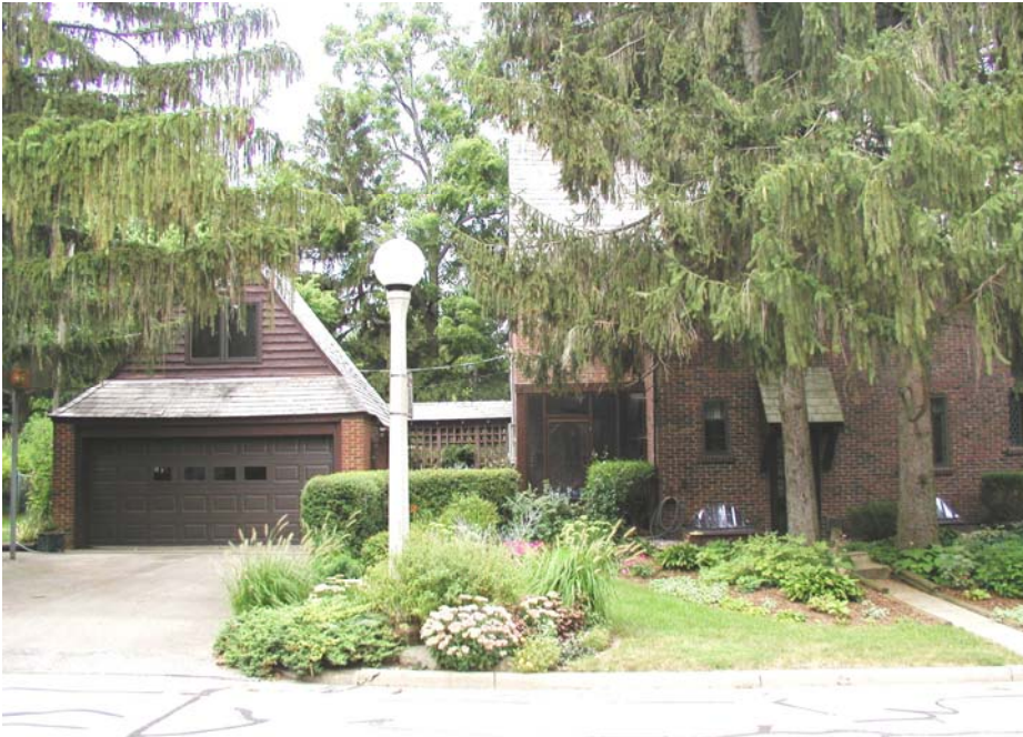
Existing garage along Carle Avenue. Proposed 3-foot addition would bring garage in line with house
