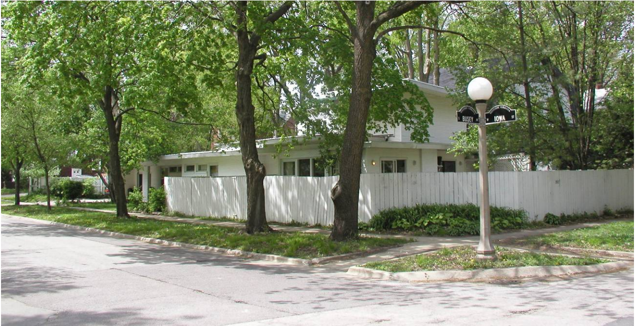
Subject property viewed from the southeast.
