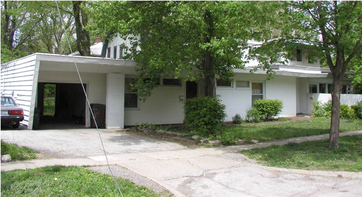
Subject property viewed from the southwest.
