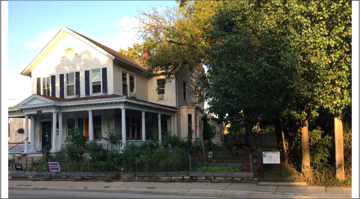
From South Cedar Street
