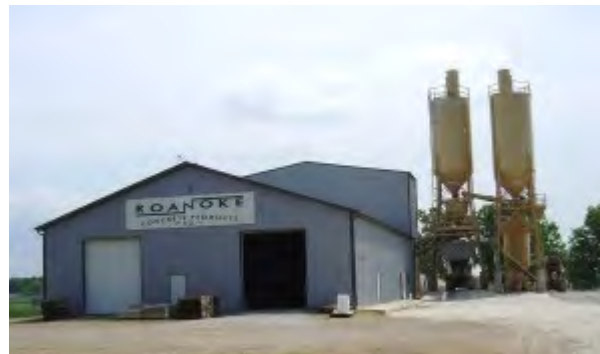
Fig. 1 – Roanoke Facility in Mossville
