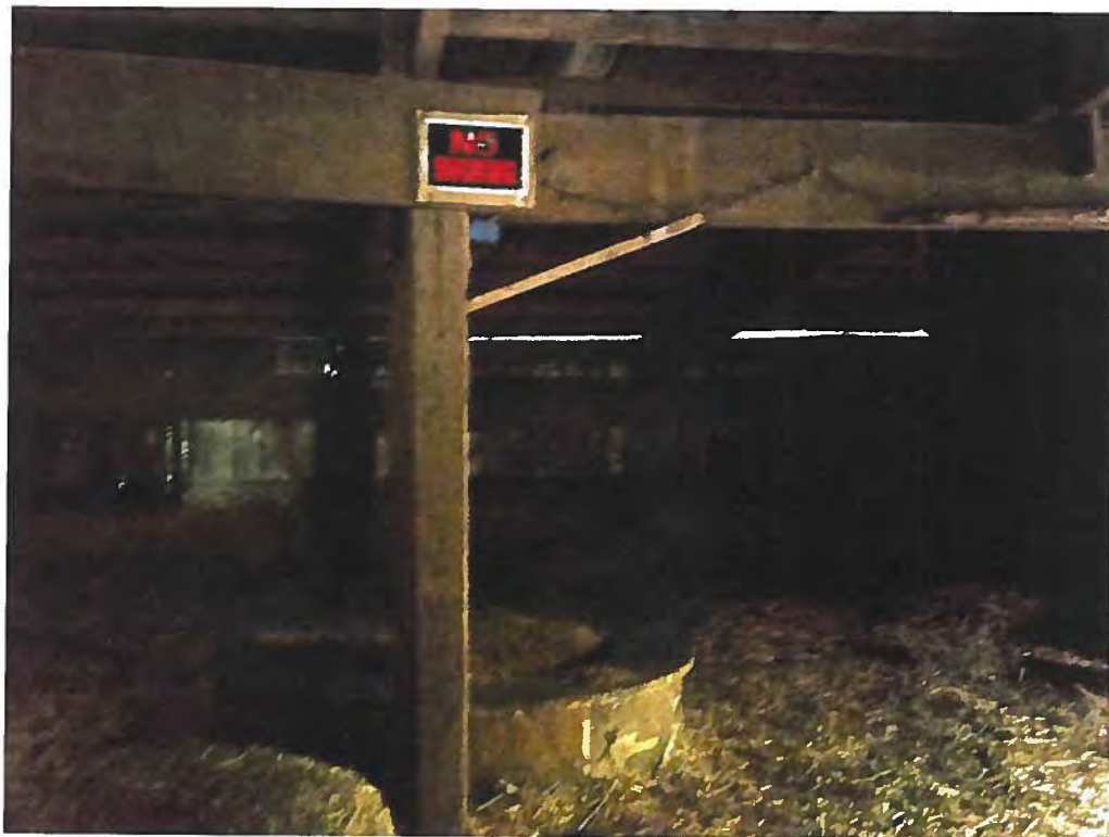
East Barn interior
