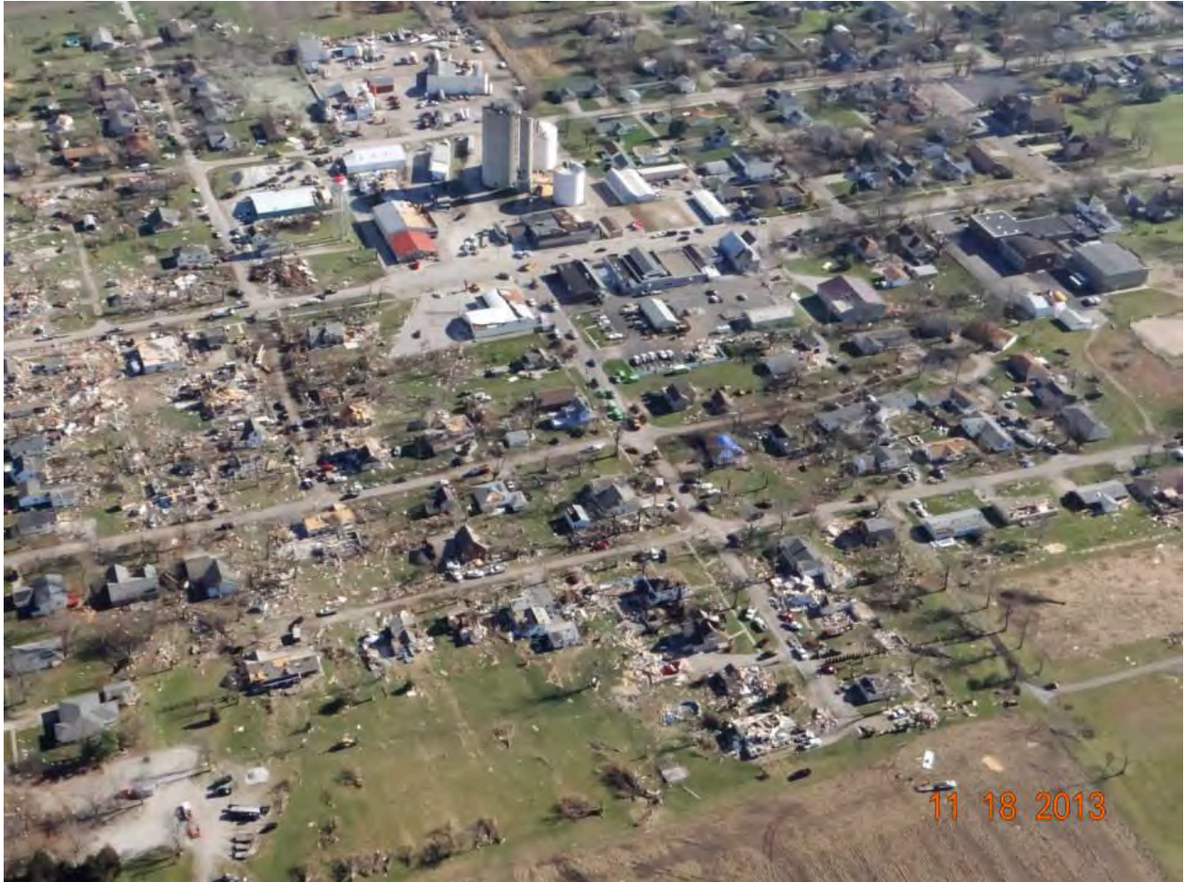
Figure 3-7. Damage to Gifford by EF-3 Tornado as Viewed on November 18, 2013
