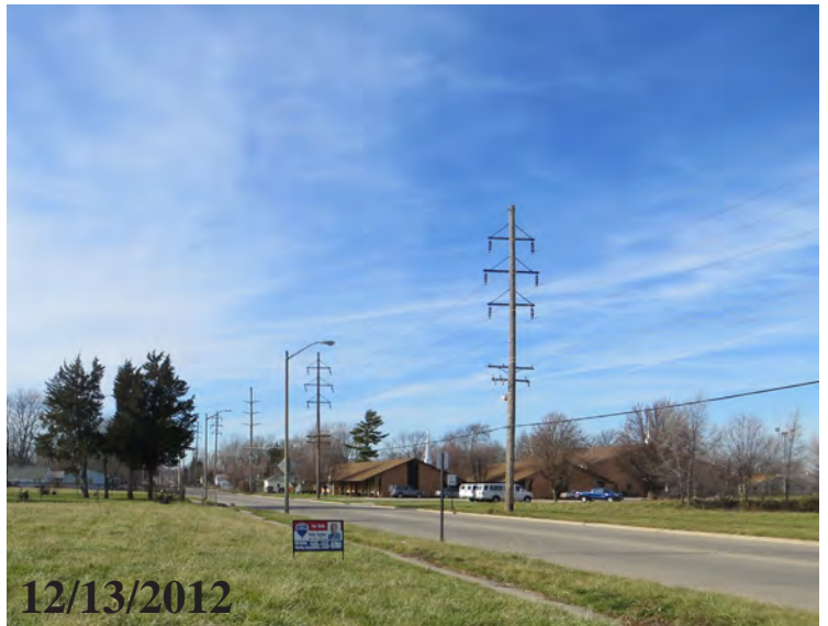
4) W Bradley Avenue - looking west towards Alpha and Omega Church
