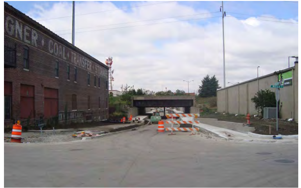
Fig. 13: Logan/Water Street reconstruction project
