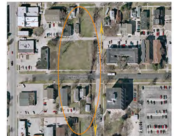
Fig. 4: Boneyard Creek site before construction
