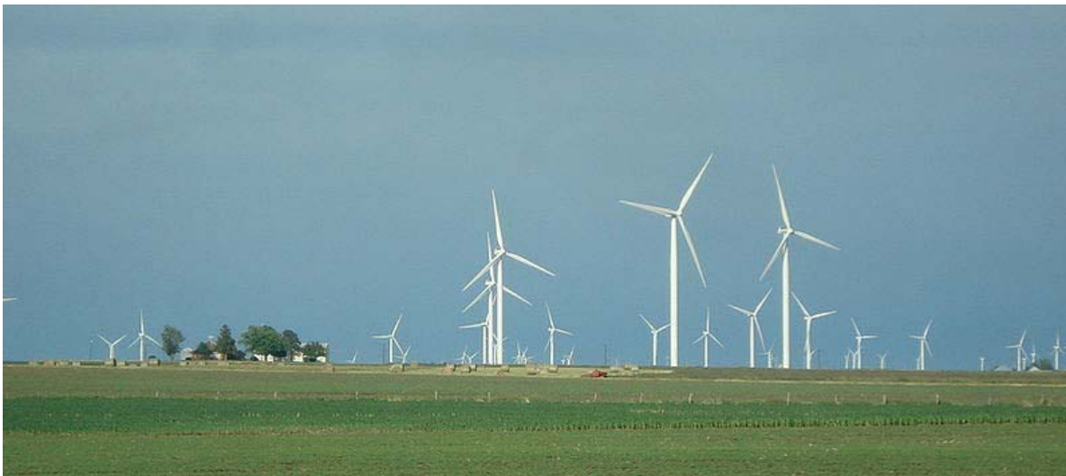
1.65 MW/269 foot rotor diameter/214 foot system height
