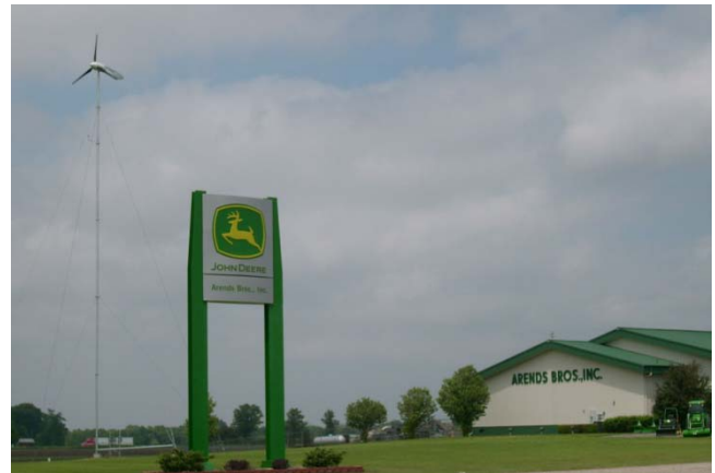
5.0 kW/21 foot rotor diameter/115.5 foot system height
