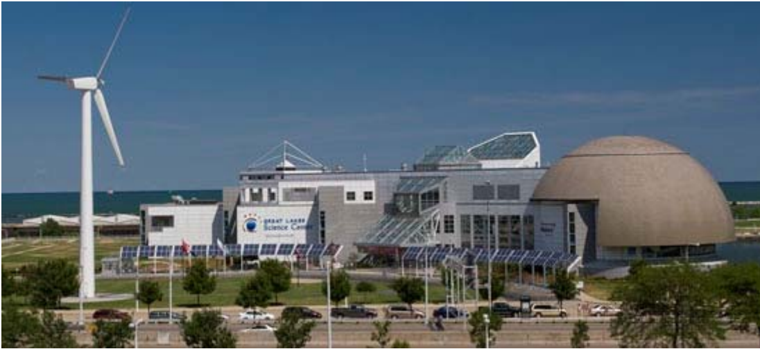
225 kW/88.6 foot rotor diameter/150 foot system height
