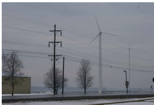
100 kW/70 foot rotor diameter/159 foot system height
