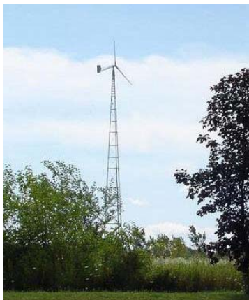
20 kW/100 foot system height
