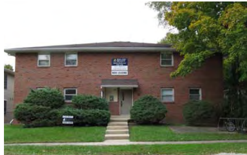
The primary entrance of this apartment building is oriented toward the street. The door hood and sidewalk focus attention on the entrance.
