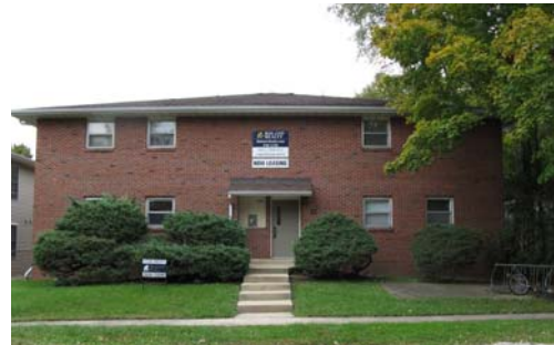
The primary entrance of this apartment building is oriented toward the street. The door hood and sidewalk focus attention on the entrance.
