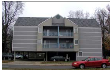
Parking on ground floor should be screened and not in the façade zone
