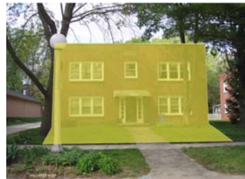
The Façade Zone is the part of the building facing a public street. Interior lots typically have one façade zone.
