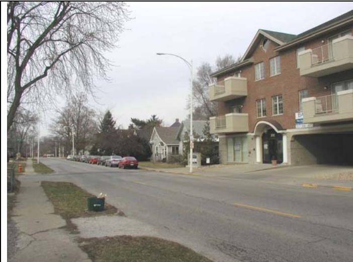
#1 - Façade and west on Springfield
