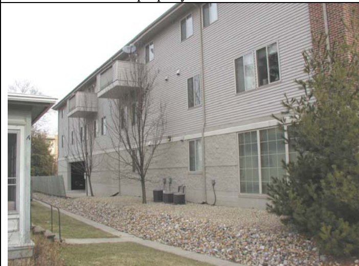
#5 - Northeast at west facade
