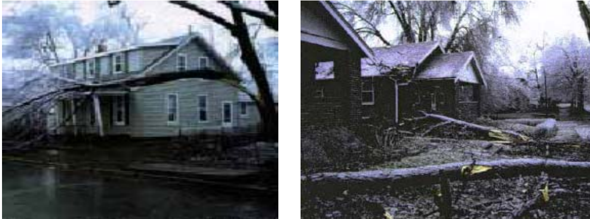
Figure 3.12 Typical Damage from Ice Storm, 1990, Urbana
