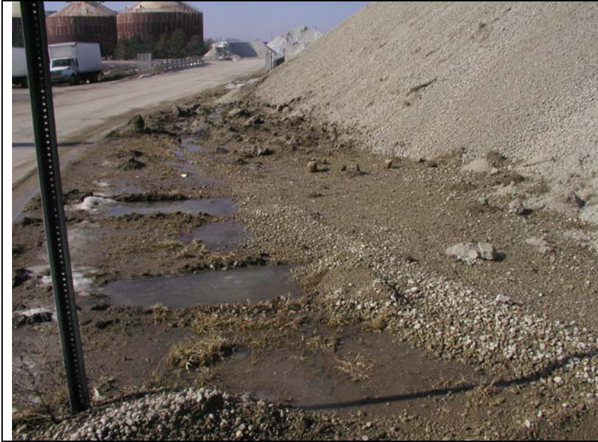
#7: West along Somer pile encroaching into City ROW
