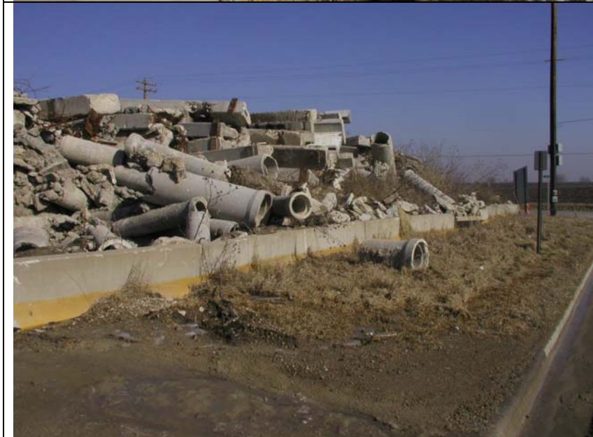
#3: Pile at corner encroachment in setback
