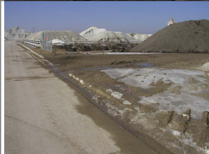
#9: View west tracks over curb and on City ROW
