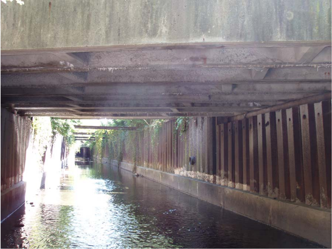
Figure 3.19 - View from McCullough Street
