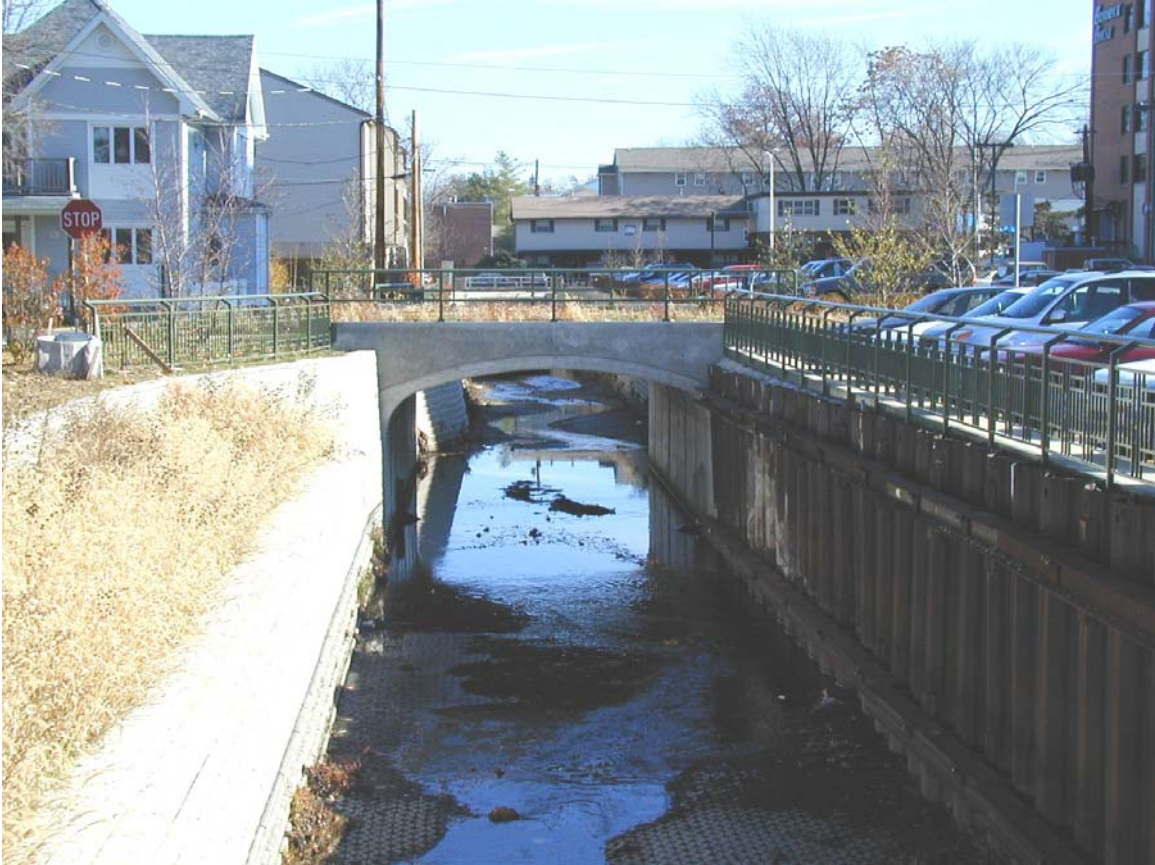
Figure 3.17 - View from Gregory Street
