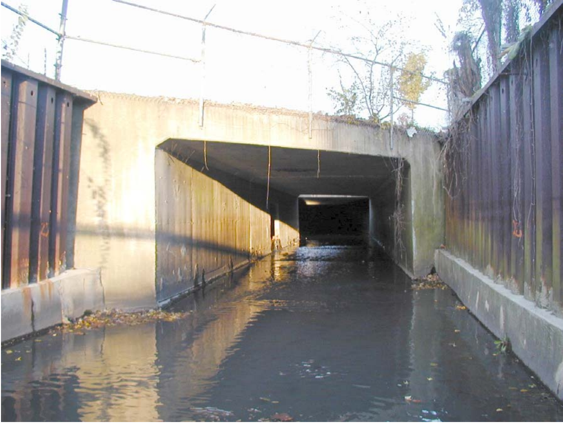
Figure 3.20 – View from Springfield Avenue
