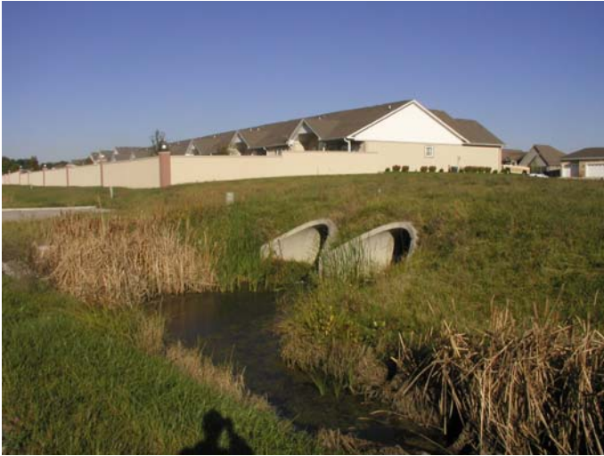
Existing two drainage pipes drainaing into ditch on U.S. Route 150.
