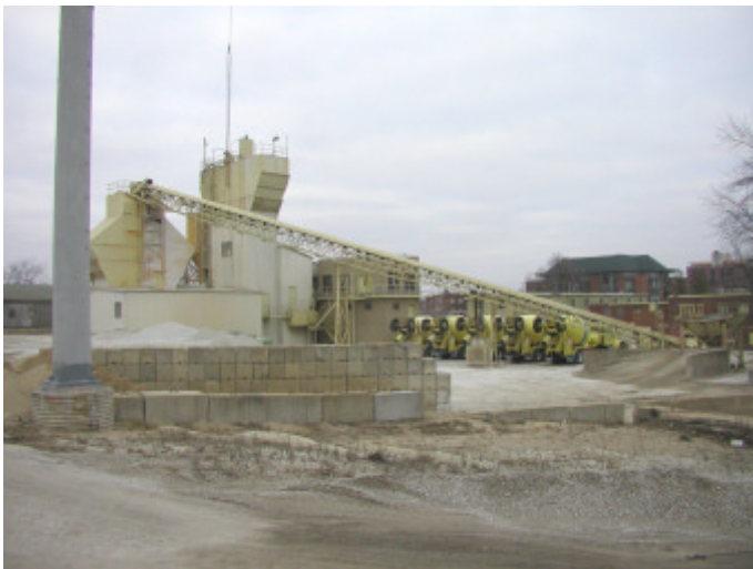
Existing Builders Supply Concrete plant on Green Street in Champaign.
