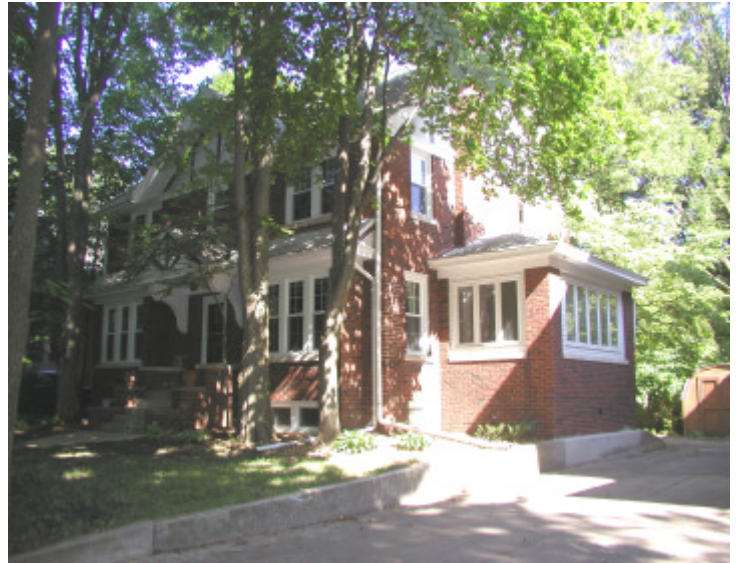
East side of property.
