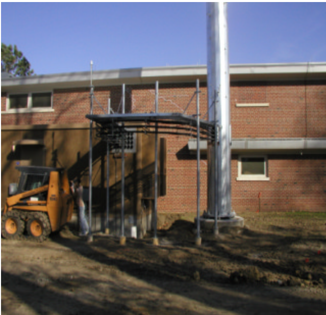
Cell Tower Site-Facing East
