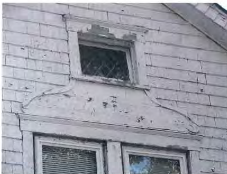
611 West Elm Street: Detail, upper window ornament, north wall
