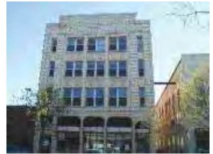
▼ Tiernan's Hall, 115 W. Main Street Built in 1871 with façade designed by Joseph Royer in 1913
