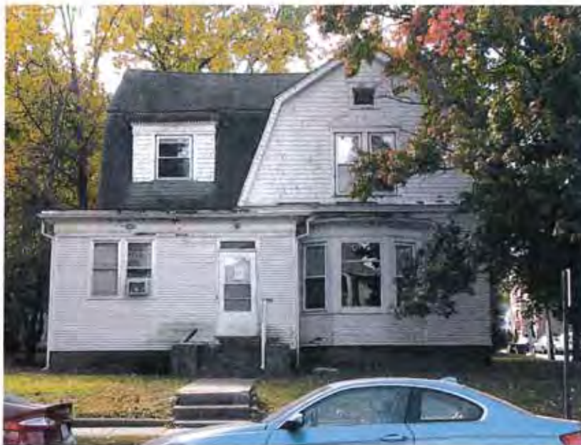
611 West Elm Street: North facade
