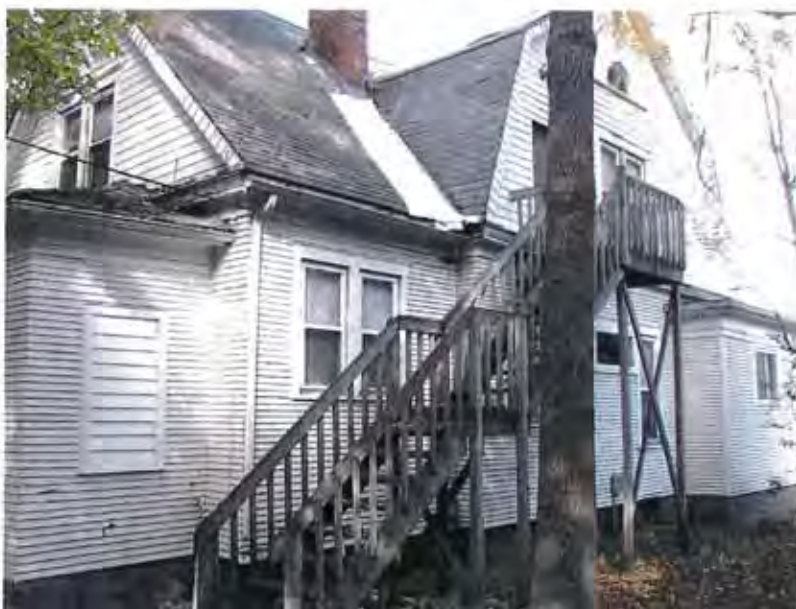
611 West Elm Street: East wall, view from southeast
