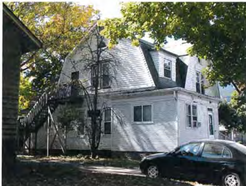
611 West Elm Street: East and north walls, view from northeast
