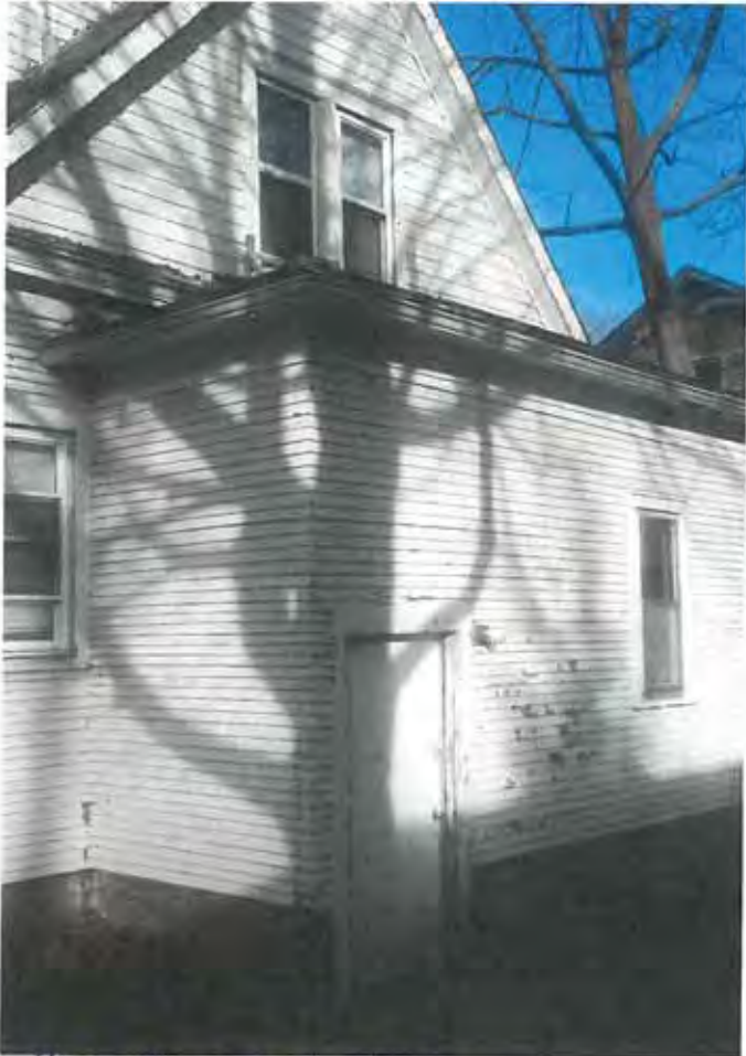
REAR PORCH MADE INTO ADDITION.
