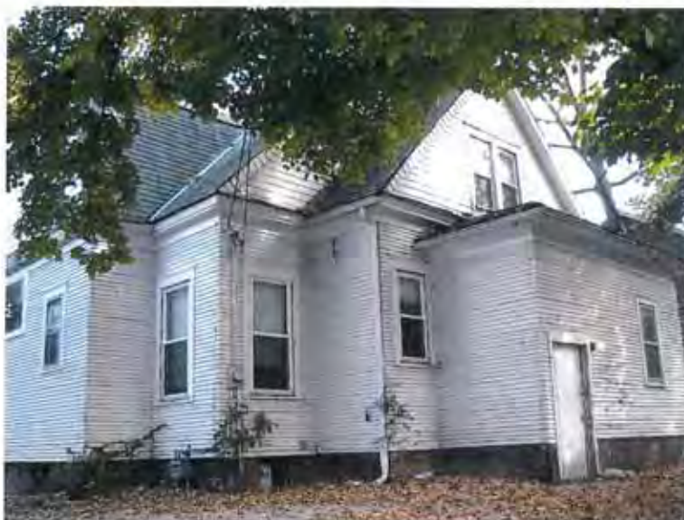
611 West Elm Street: South walls, view from southwest
