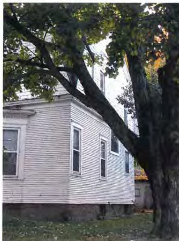
611 West Elm Street: West wall
