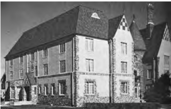
Zeta Tau Alpha House Addition Completion, 1963
