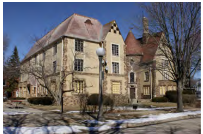
Zeta Tau Alpha House Addition, 2013
