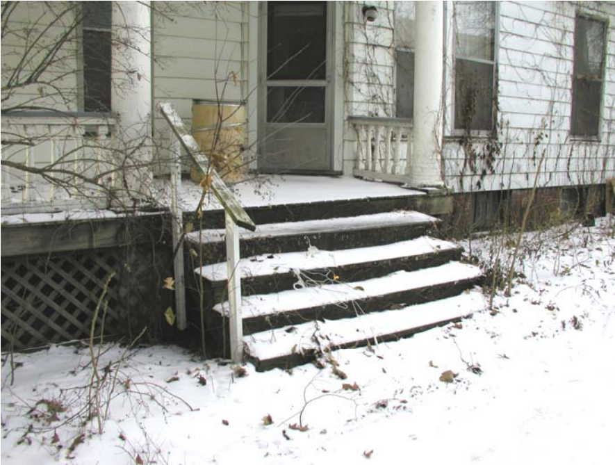
East Façade Porch Stairs
