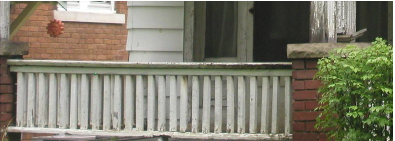
Detail of the railing
