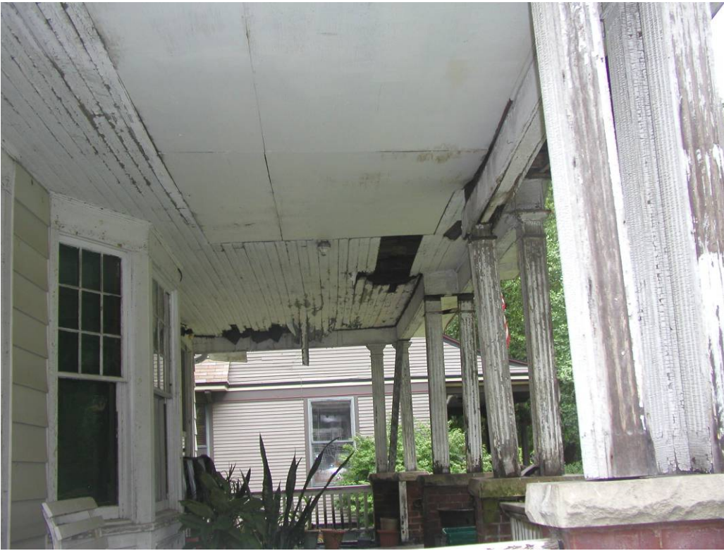
The ceiling appears to have been patched with plywood
