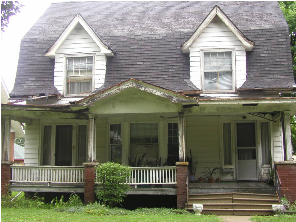
The original porch before demolition
