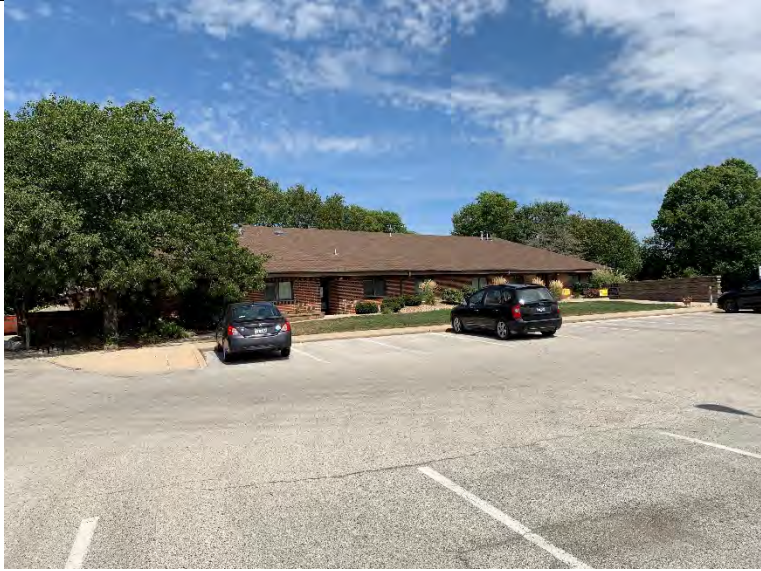
Figure 1. Looking northeast across parking lot towards Main Building.
