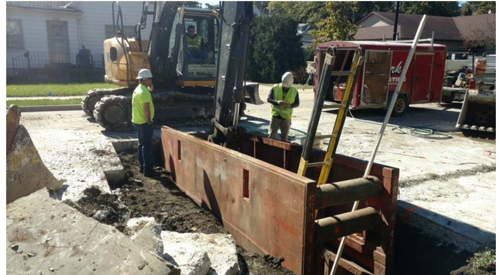
Construction of Sanitary Sewer Extension Along Springfield Avenue
