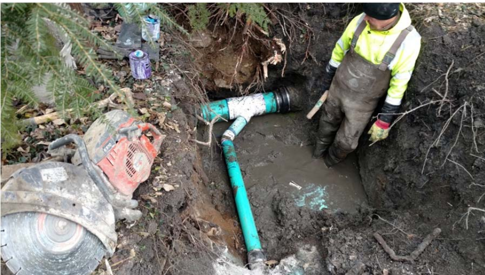
Miscellaneous Sewer Repair Project
