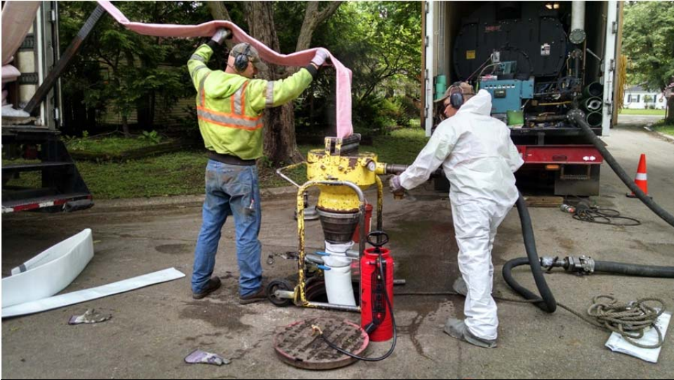
Cured-In-Place Pipe (CIPP) Rehabilitation
