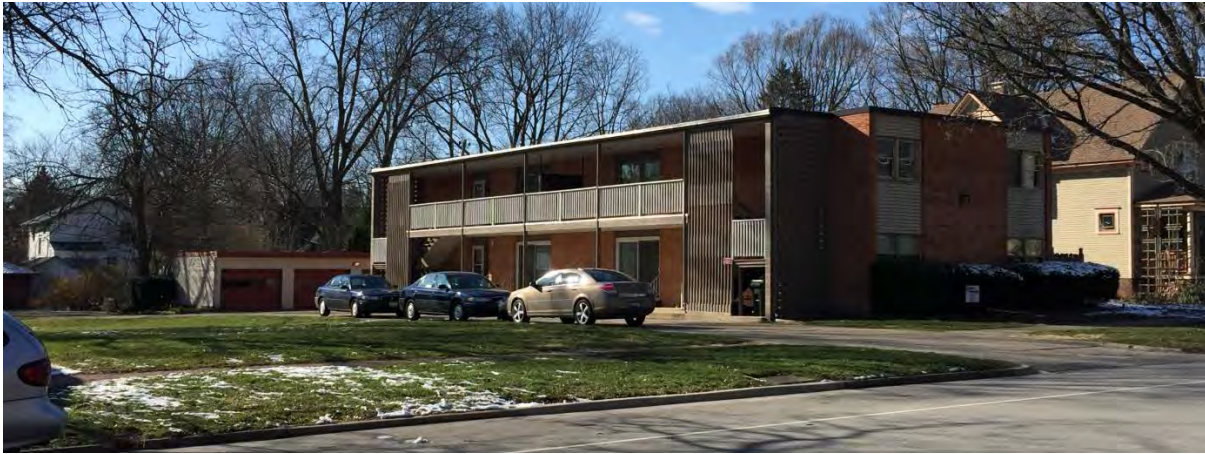
Figure 1. Dwelling and garage at 717 S. Broadway Ave.
