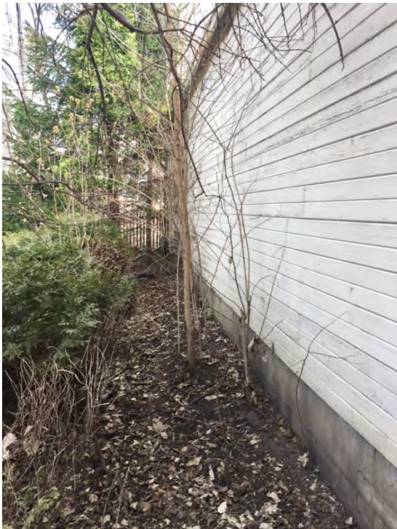
Figure 3. Rear yard: 36" between garage and bushes.
