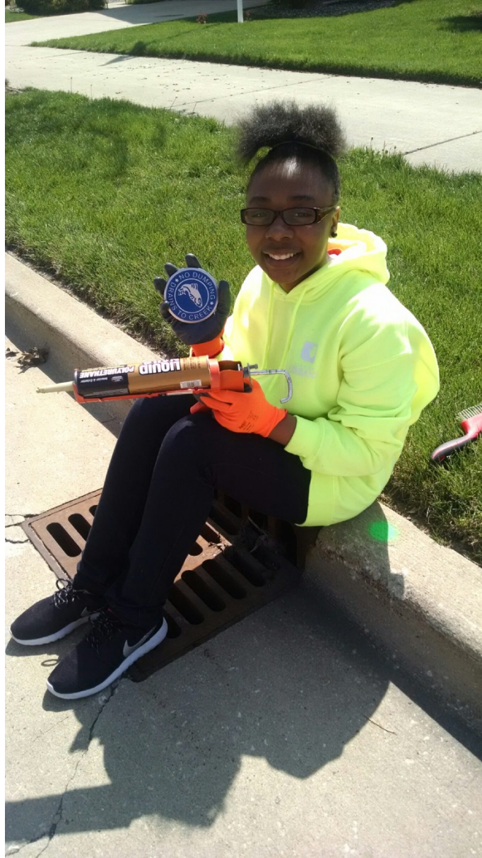
Photo of Storm Sewer Medallion Installation
