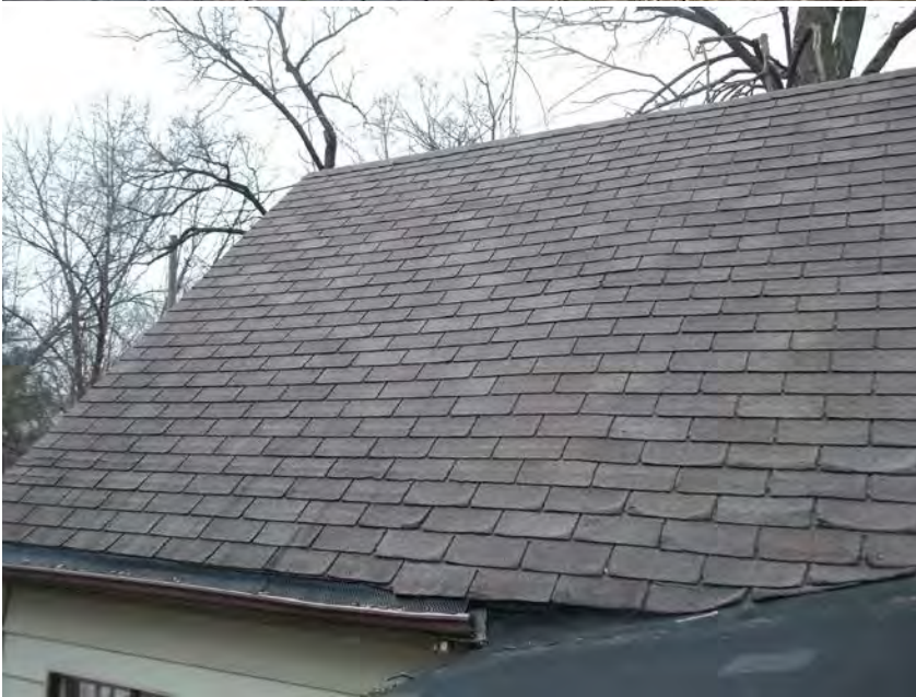
South Gable East Face
