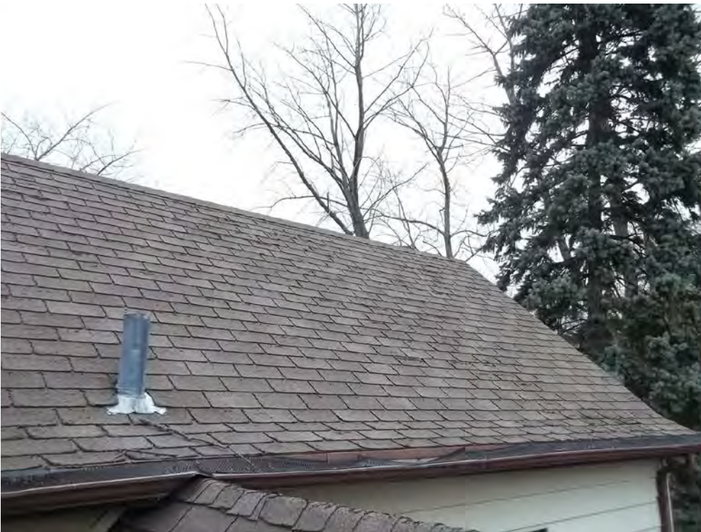
East Gable South Face
