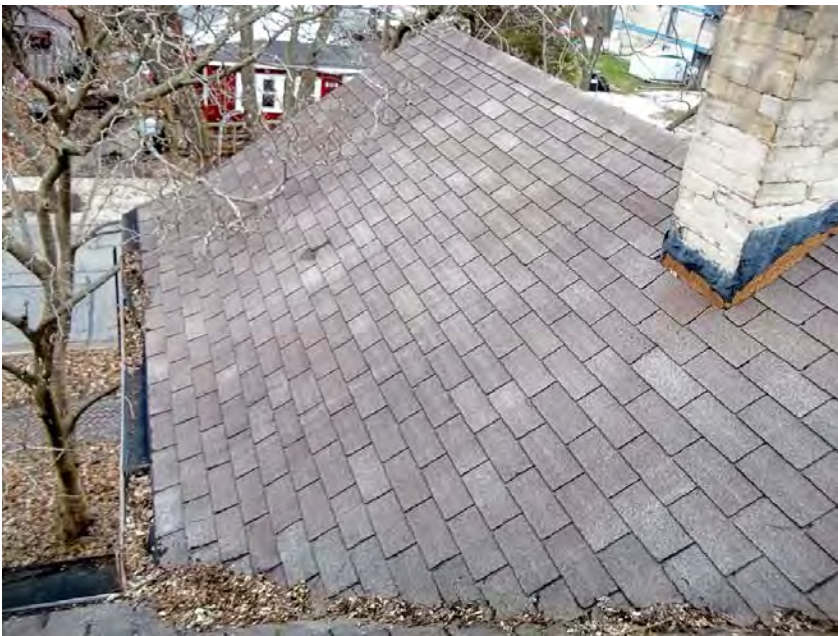
North Gable West Face
