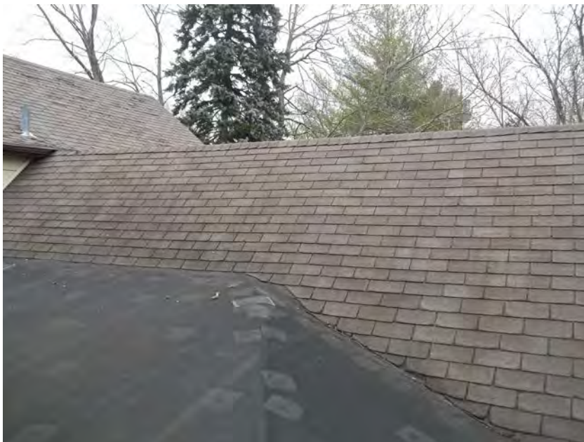
South Gable West Face (1st)
