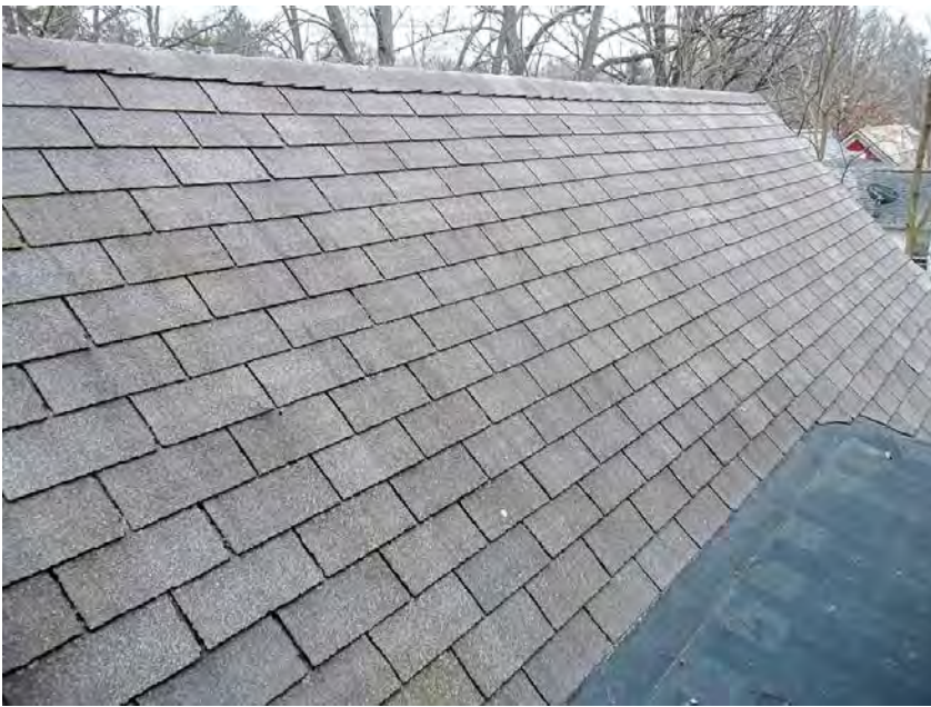
South Gable West Face (2nd)
