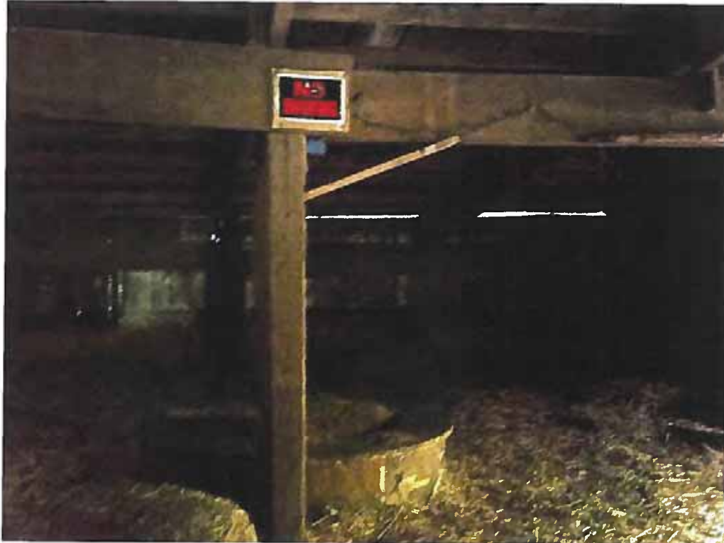
East Barn interior
