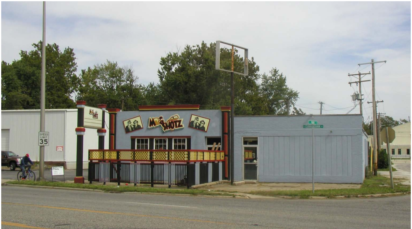
View from the west. The proposed canopy will be located where the current wall signs are.
