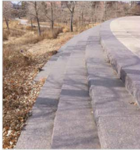
<DESCRIPTION> AT CREEK EDGE: 12" THICK, VARIED LENGTH, VARIED WIDTH AT STONE BLOCK BENCH: APPROX 18" HEIGHT, VARIED LENGTH
