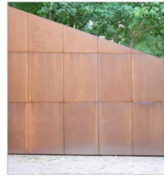
<DESCRIPTION> NON-STRUCTURAL STEEL PANEL FASTENED TO A STRUCTURAL SHEET PILE WALL
