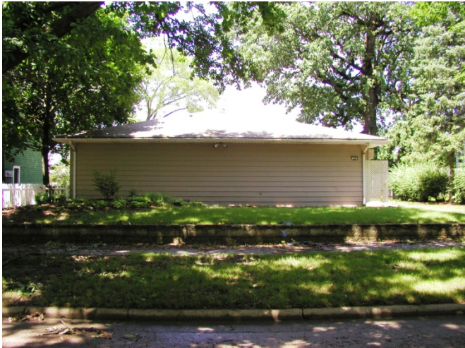
Figure 2. 506 East Elm Street – front façade
