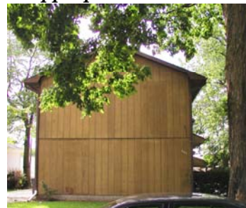
This apartment building is sided with wood, a quality material, but faces sideways instead of facing front. The façade of the building is blank, which can have a negative impact on the neighborhood.
