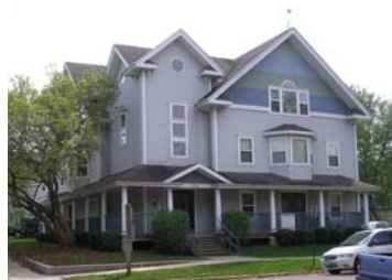
The doors, windows, and trim are interesting details.
