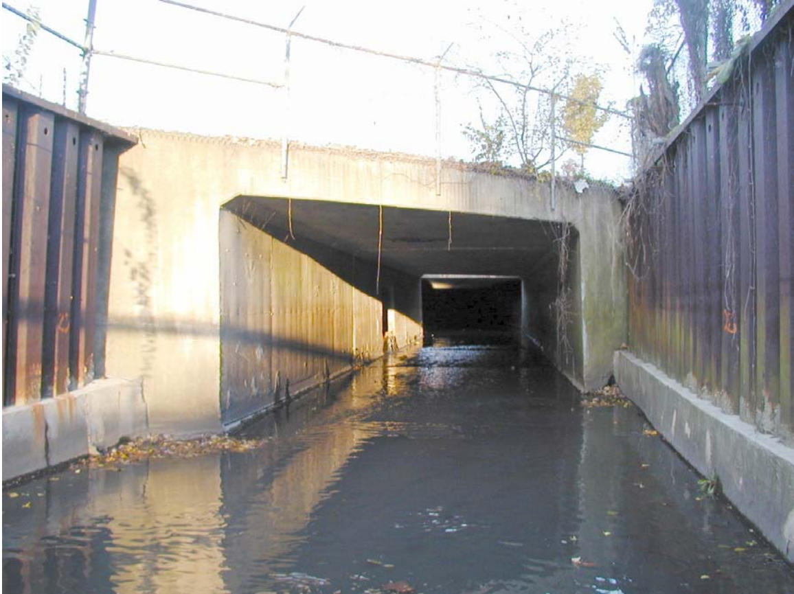
Figure 3.22 – View from Springfield Avenue
