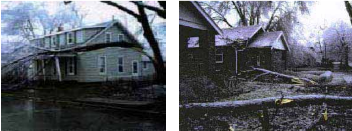
Figure 3.12 Typical Damage from Ice Storm, 1990, Urbana
