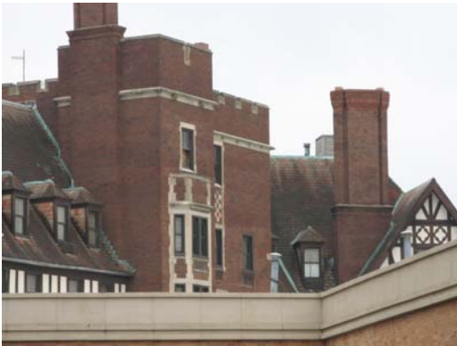
Another view of south façade
