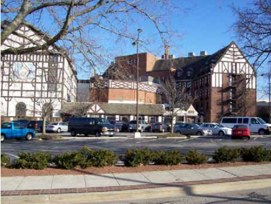
Urbana Lincoln Hotel: Current west entrance
