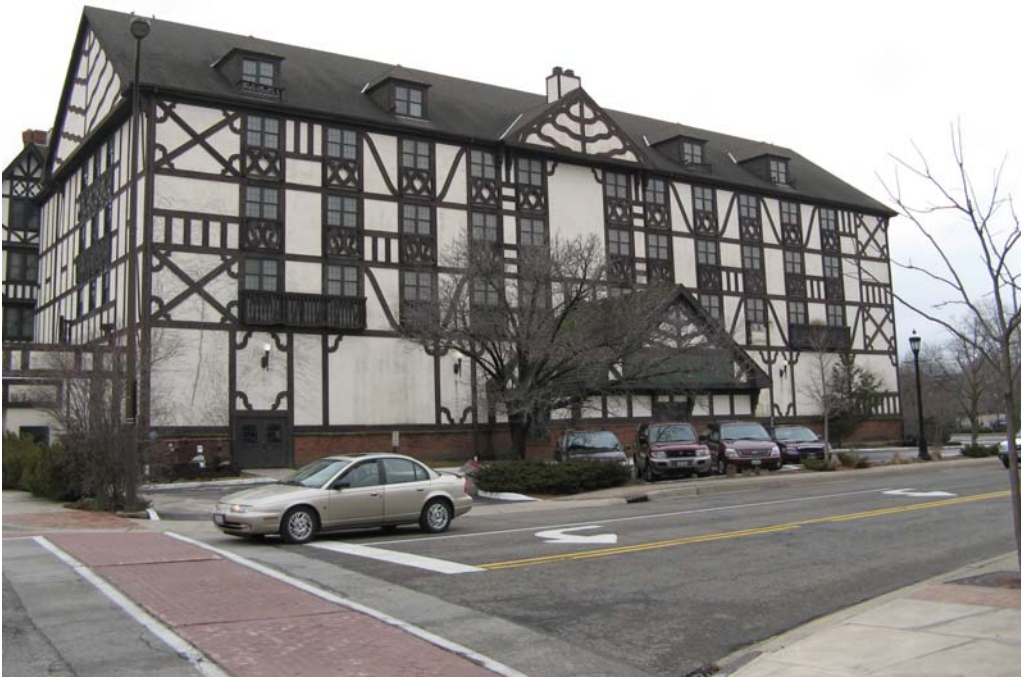
North façade, nearly entirely 1980s addition
