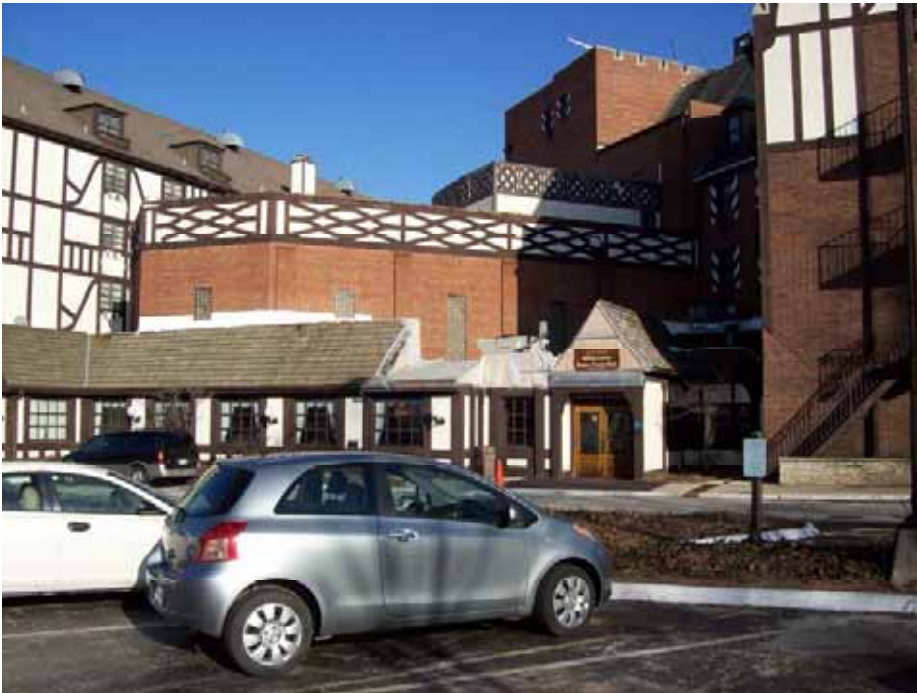
Urbana Lincoln Hotel: Current west entrance (detail)
