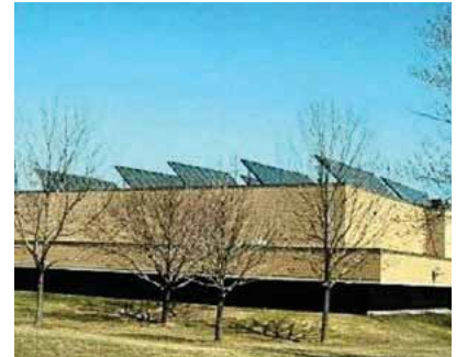
Solar panel installation.
