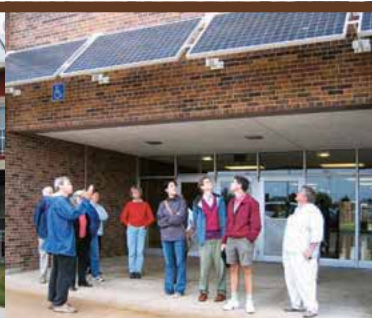
Solar electric awning on Memorial High School, Madison, Wisconsin.
