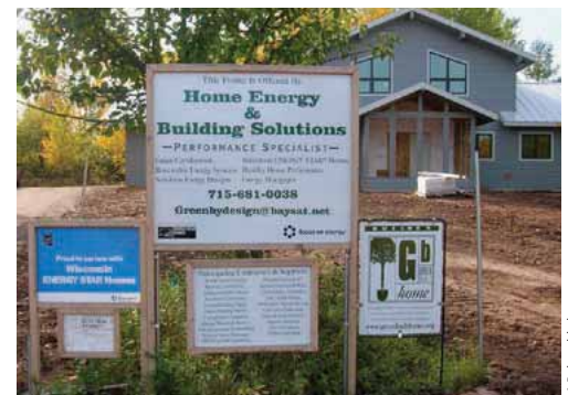
An increasing number of local builders and organizations in Wisconsin are providing green building and energy services.
