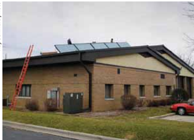
City of Madison fire station solar thermal panel installation.
