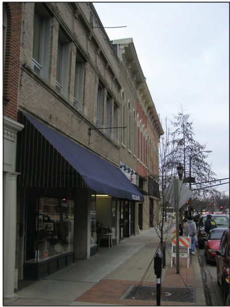
Main Street, looking east
