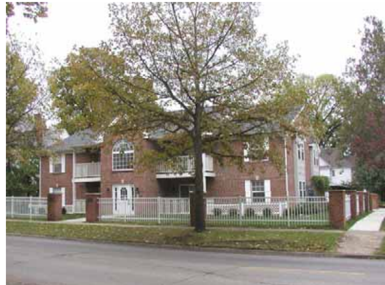
611 W. Green. A multi-family residence was replaced with a new multi-family residence.
