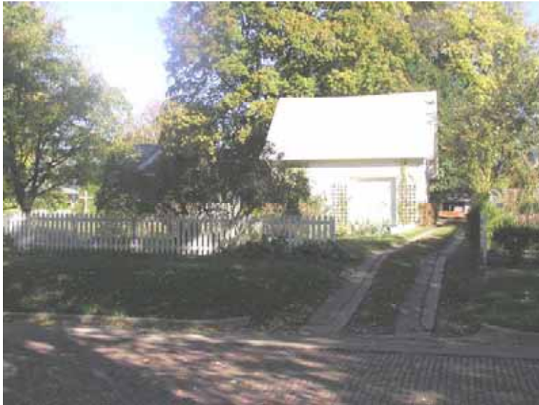
606 W. High. The lot has become an extended yard.
