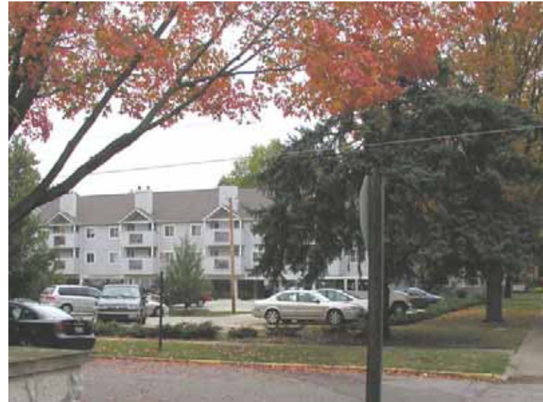
508 & 510 W. Green. Parking for the Presbyterian Church.
