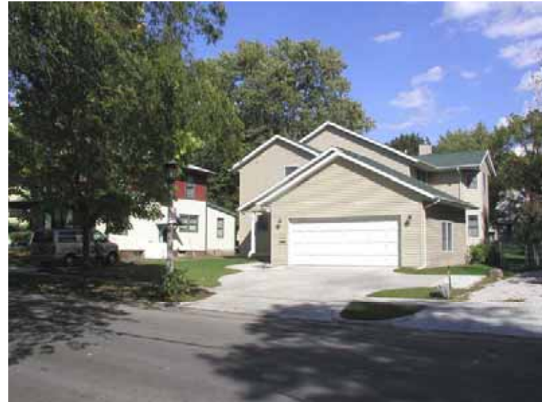
708 Race. A single family home replaced the demolished home.
