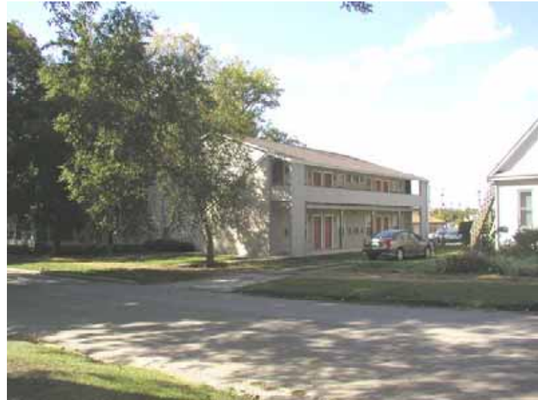
406 E. Elm St. An apartment Building.
