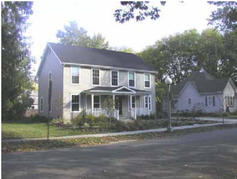
208 W. Oregon. A single-family home replaced the demolished home
