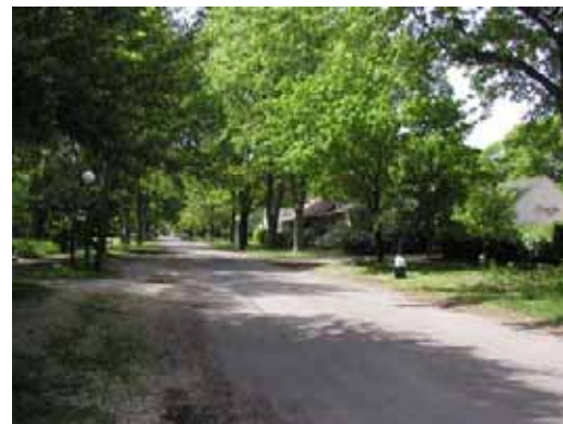
Figure 7. Not all streets have curb and gutter system.
