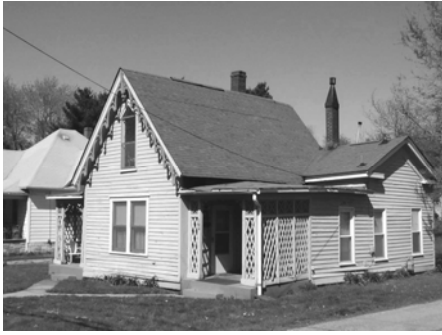
Gothic Revival Cottage
