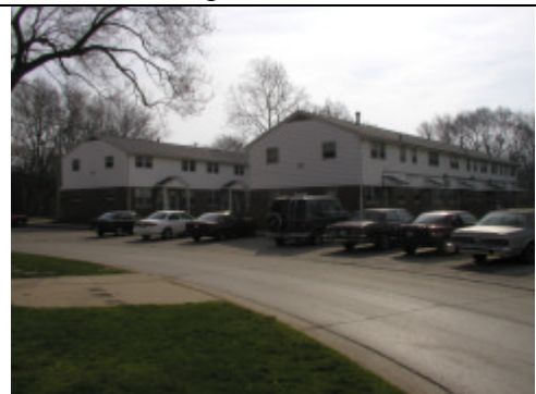
F. Lakeside Terrace @ bend facing Southeast.
