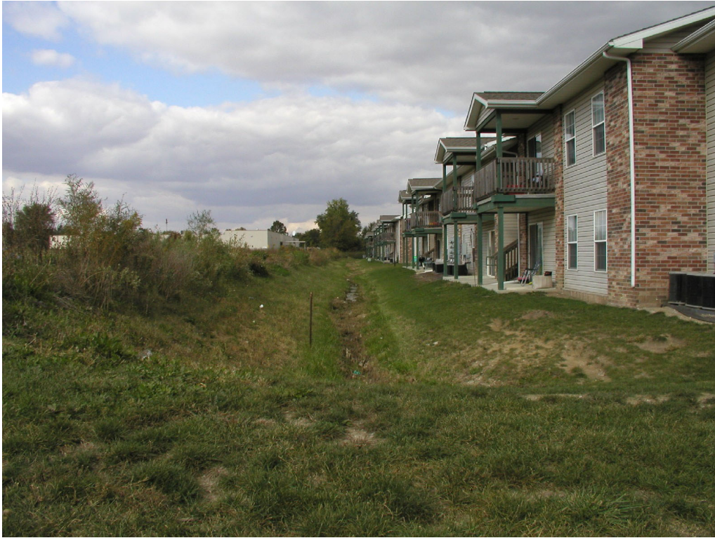
Photo of drainage swale
