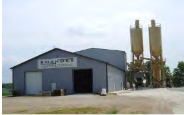
Fig. 1 – Roanoke Facility in Mossville
