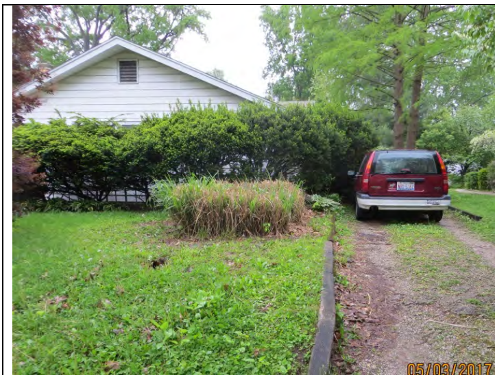
Figure 1. 613 W. Washington facing south
