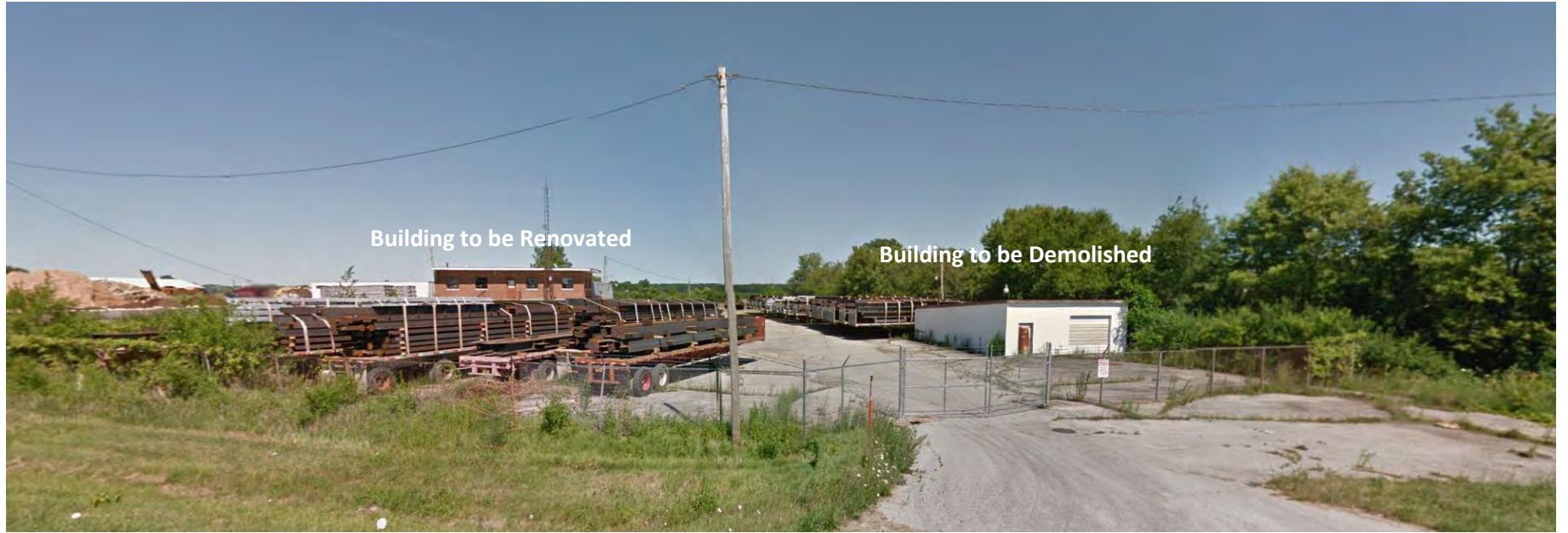
Exhibit D: Site Photo, Looking East
