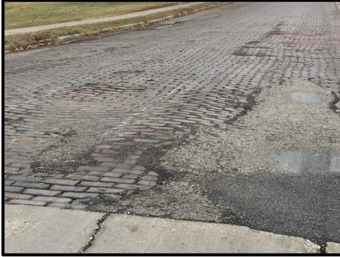
Photo 1: Asphalt Patch Used To Correct Rutting
